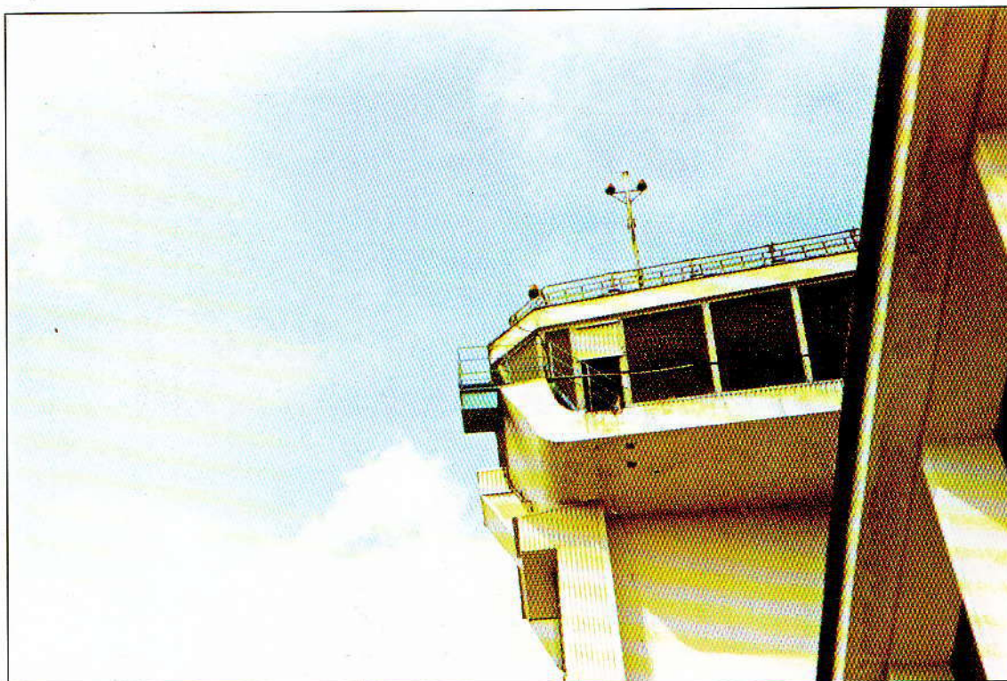
Air traffic control Tower Warsaw airport Poland
